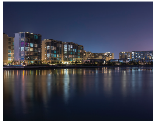
There were foundation pours of over 3,000m 3 .
