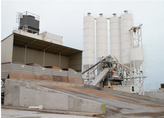
➤ Readymix Abu Dhabi has invested heavily in the latest plant and equipment.
