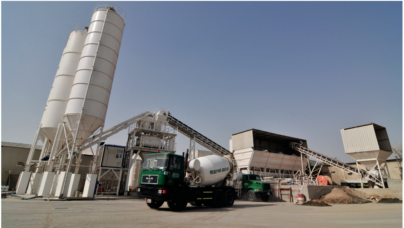
Readymix Abu Dhabi's Al Ain batching plant - certified by the National Ready Mixed Concrete Association (NRMCA) and calibrated by Bureau VERITAS.
